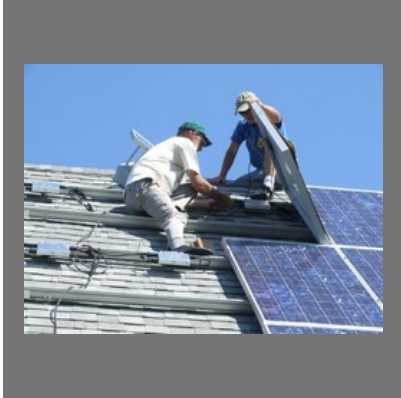
Solar Panel Installation
