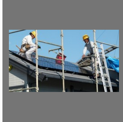
Solar Roof Top System Installation
